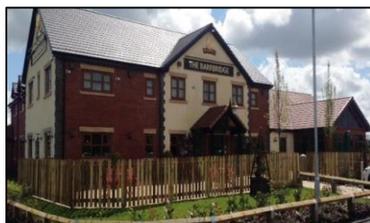
'The Barrbridge', Coatbridge
